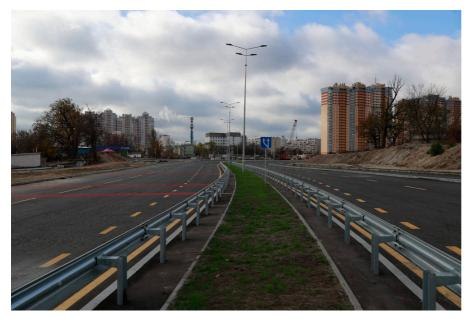
Kyiv mayor Vitali Klitschko visited Velyka Kiltseva ring road to see newly constructed road section between Rokossovsky av. and Sim'i Kulzhenkiv street. The road has already opened to traffic. Construction project includes: asphalt paving, kerbs, storm water drainage, LED street lighting, pedestrian overpasses and landscaped sidewalks.
